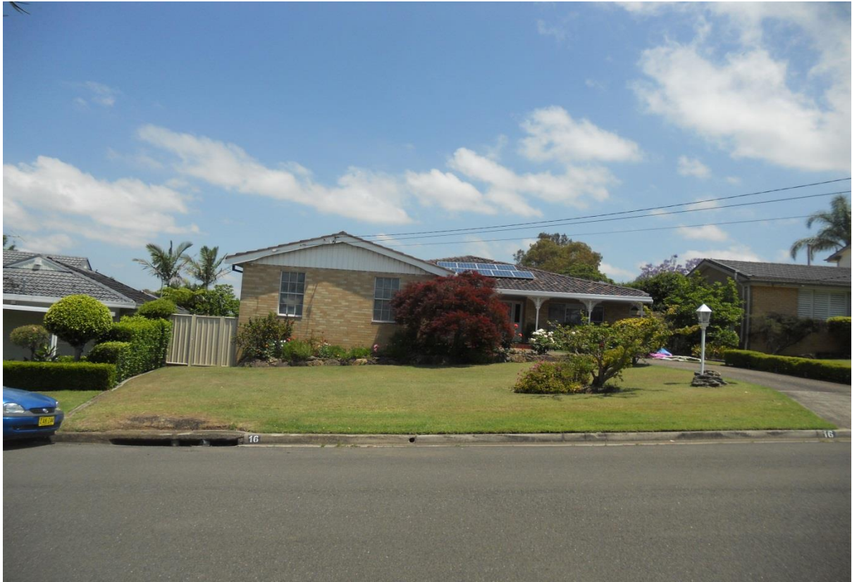
Figure 7 View South Towards 16 Kay Street (Dwelling at Rear of Subject Site)
