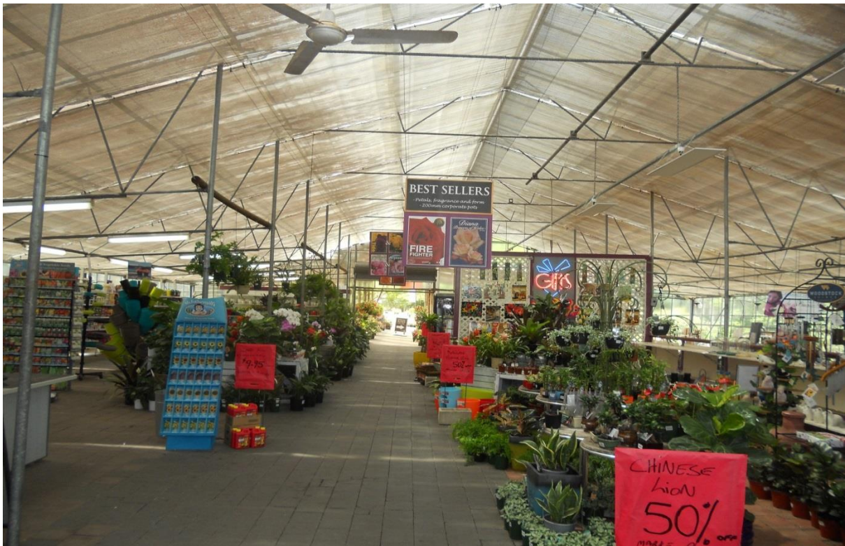
Figure 21 View Inside of Retail Centre of Swane's Nursery
