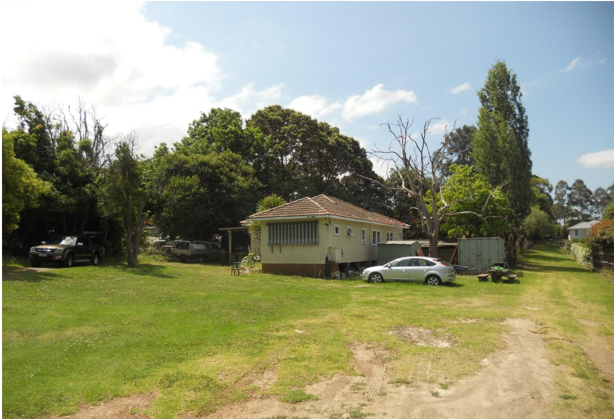
Figure 5 View North Towards 235 Marsden Road (Swane's Nursery) Unsealed Access Handle to St Pauls Anglican Church Cemetery on Right
