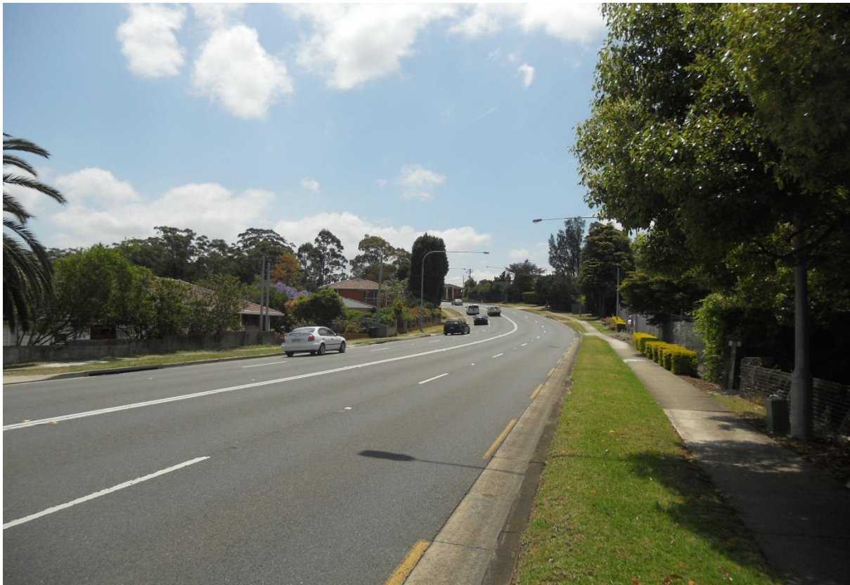
Figure 10 View North-West Along The Streetscape of Marsden Road
